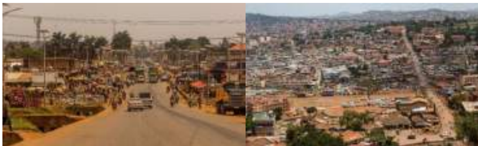
Figure 20-21. Kampala city roads and buildings. In the city center, the primary pathways consist of concrete-asphalt, whereas the secondary pathways are composed of compacted dirt; in the suburbs, all pathways are entirely compacted soil. Open drainage ditches alongside concrete and asphalt main roadways facilitate swift water release during tropical rainstorms (Erdem, 2024).
