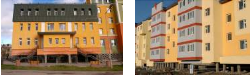
Figure 8-9. Buildings built on piles to protect the permafrost zone (Yamata, 2002-2007)
