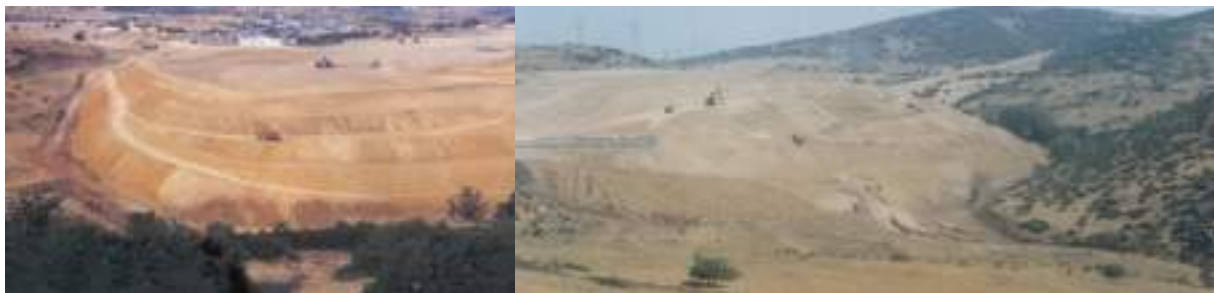
Figure 4. The first stage of rehabilitation with soil cover at Environmental Park of Derveni. (Photos from FODSAKM archive)
