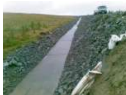
Figure 13-14. Open roadside drainage ditches in the suburbs (Yamata, 2002-2007).
