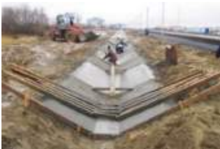
Figure 13-14. Open roadside drainage ditches in the suburbs (Yamata, 2002-2007).
