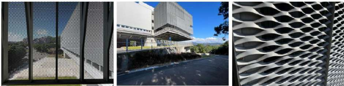
Figure 5. The expanded metal mesh's Interior, exterior, and details. (Source: Photographed for this study)
