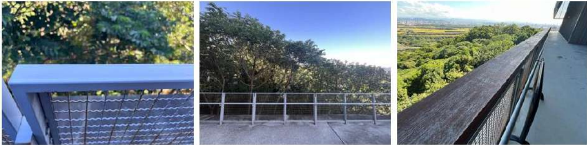
Figure 6-1. Second-floor railing; Figure 6-2. Third-floor railing. (Source: Photographed for this study).
