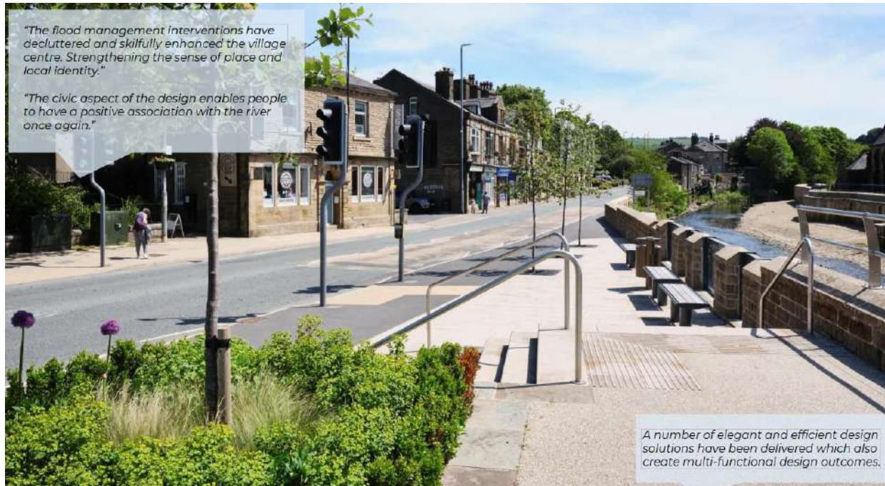
Figure 3. Mytholmroyd's completed flood defence works creating new public realm
