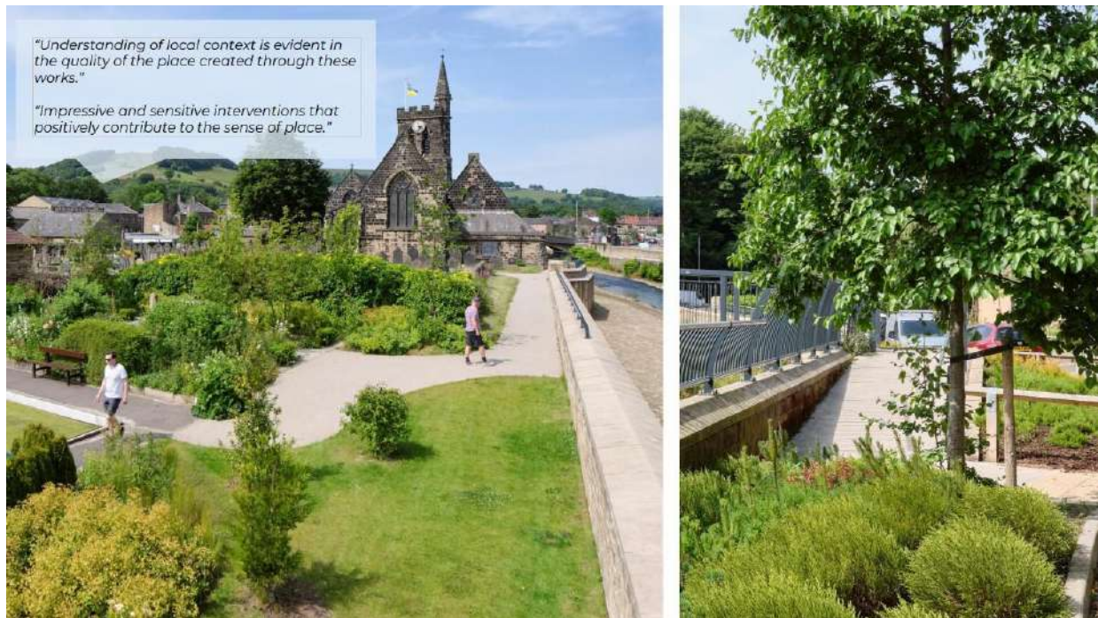
Figure 4. Mytholmroyd flood defence interventions : Atkinsrealis photography 2023
